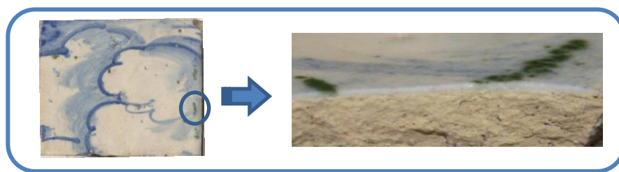
Fig. 1: Detail of the green deterioration marks present in the ceramic tiles from the panel “The Great View of Lisbon”.
